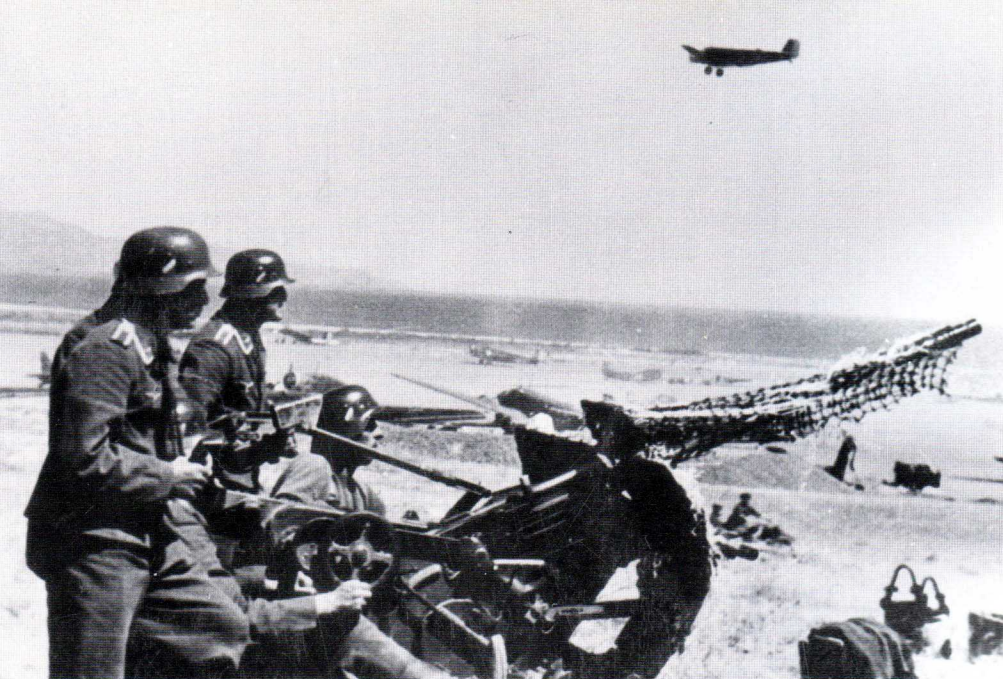
above: Once they had captured Maleme aerodrome, the Germans brought in light AA defence, such as this 2cm Flak 30. Introduced in 1935, it had a maximum effective ceiling of 7,200ft and a rate of fire of 120rpm. Alexander Turnbull Library — DA11983
