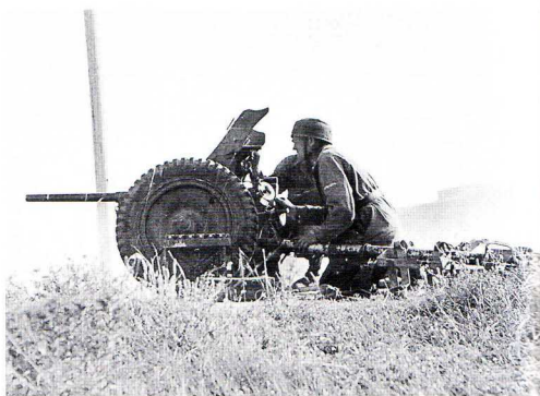
Above: A 3.7cm Pak 35/36 L/45 anti-tank gun in action. Of all the German anti-tank guns used during World War 2 this was the most widely encountered. Using AP40 ammunition it could penetrate 49mm of armour at 400yds. B. L. Davis Collection
